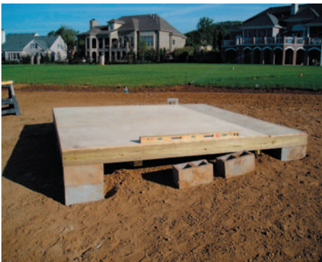
Foundation set on site
