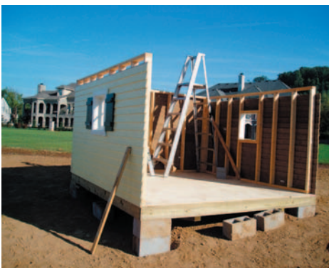
Sections assembled on foundation
